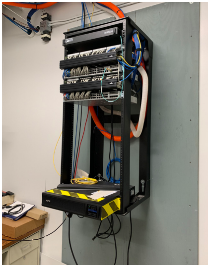
In this TR, the wall-mount open rack is mounted on properly treated, standards-compliant plywood.
