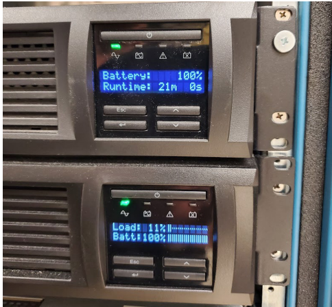
These two standards-compliant rack-mounted UPS units display adequate battery life and run times.
