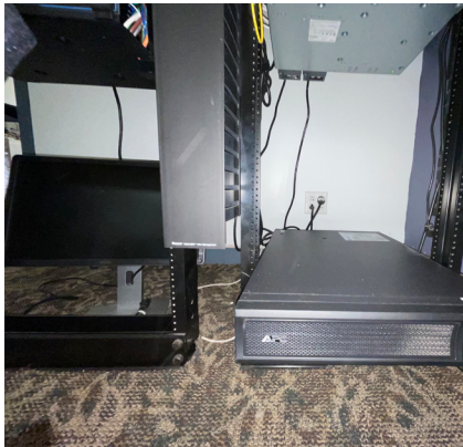
Carpeting is not a standards-compliant flooring type due to risk of ESD.
