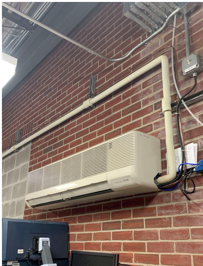
TRs require a dedicated Air Conditioning unit with independent controls. The split unit shown here works well for the space.
