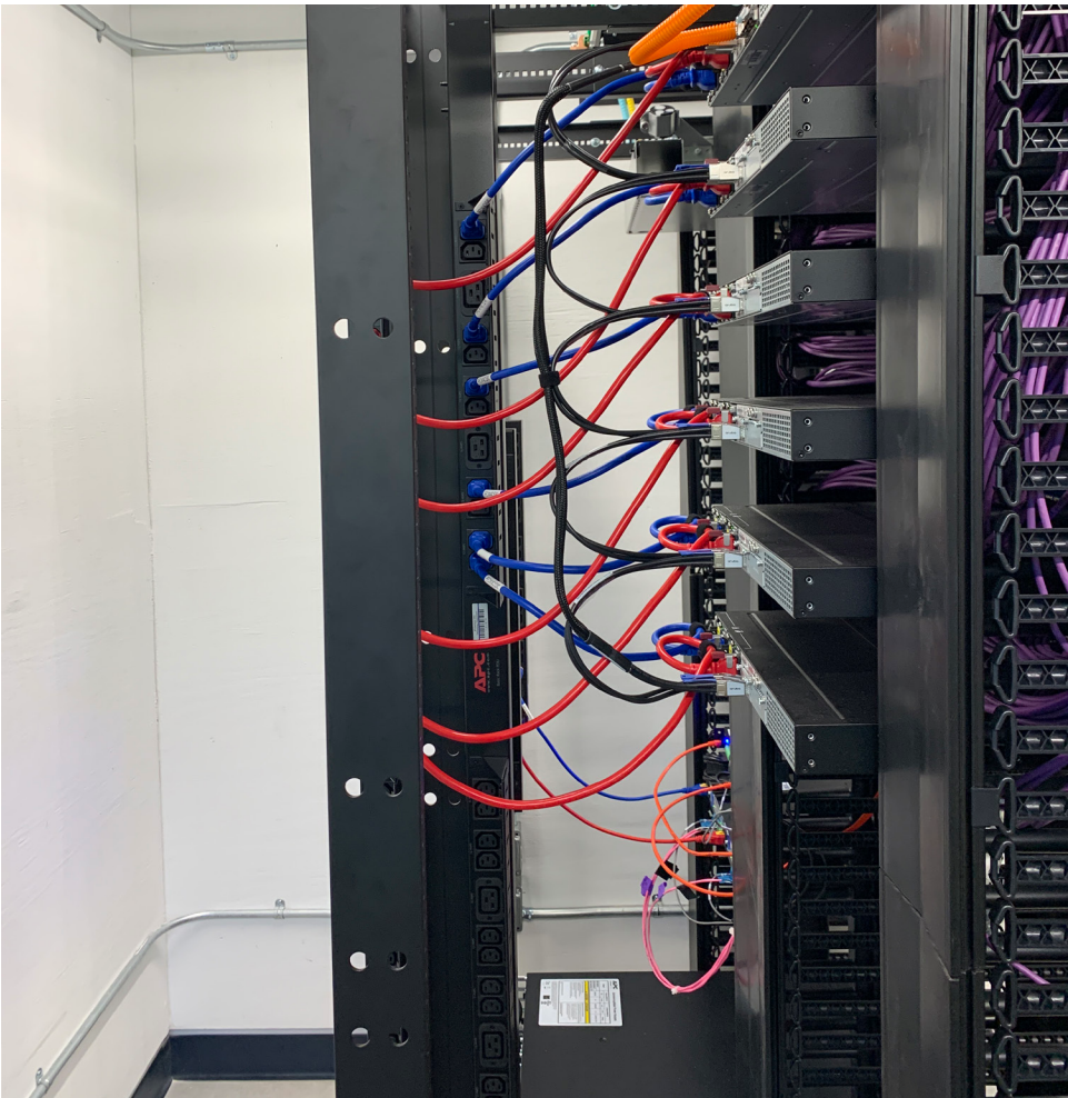
In this TR, the wall-mount open rack is mounted on properly treated, standards-compliant plywood.
