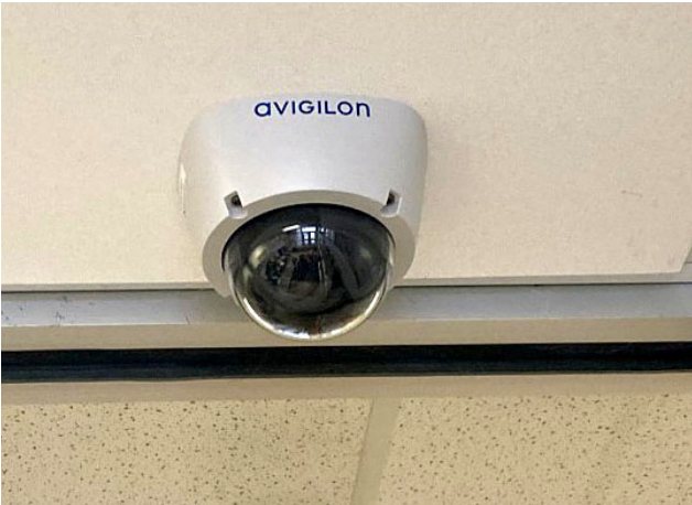
A ceiling-mounted surveillance camera can provide good security coverage of the front of the equipment rack in the space that is installed near the opposite wall.
