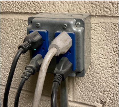
While a TR emergency power outlet is present and in use, it is not properly labeled.
