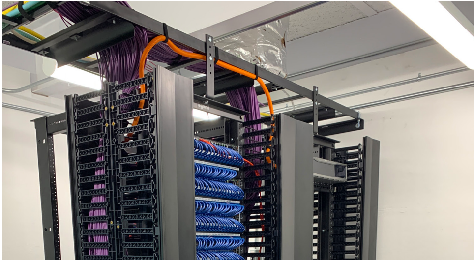
A standards-compliant ceiling open to the deck to improve air circulation.
