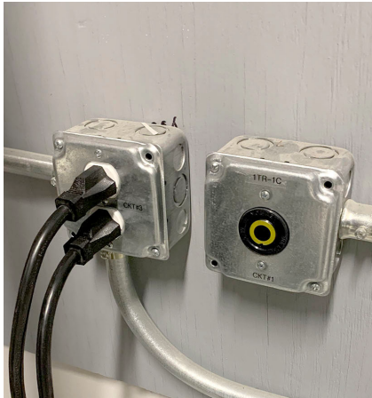
A dedicated electrical circuit with (2) 20A outlets (left) and a higher amperage twist-lock usually used for powering UPSs.
