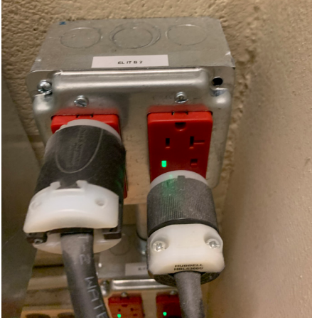
These emergency power outlets are correctly labeled and used in this TR.
