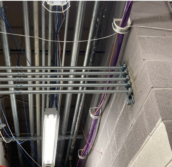
J-hooks can be used for proper support where cables exit the tray and transition to conduit in areas with inaccessible ceilings. J-hooks are used here to support the Cat cables at right.
