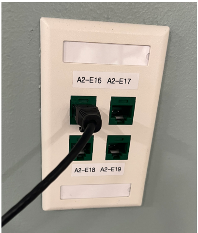
Whenever possible, data outlets shall be flush mounted. Labels shall be machine printed and not hand written.
