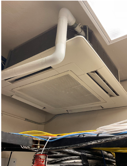
HVAC equipment must not be installed directly over a rack as it presents a water threat to the IT equipment.
