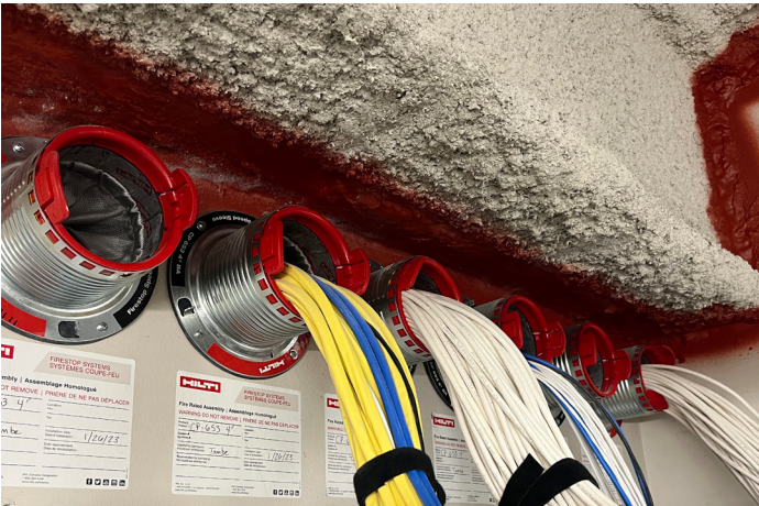
Below: Standards-compliant, fire-rated wall penetration assemblies.
