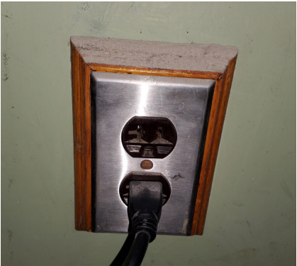
This outlet is not dedicated and lacks both emergency power and proper labeling.
