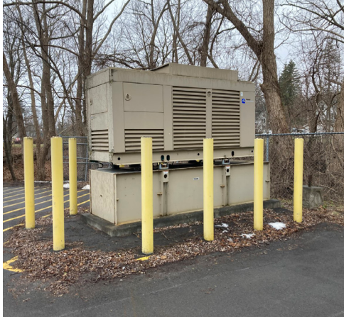
Building generators provide electrical power to connected outlets installed throughout the facility including in all TRs.
