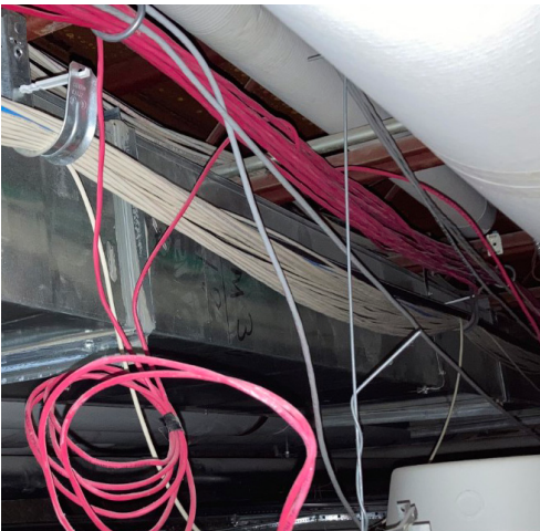
J hooks be spaced 4' apart and staggered 2 – 3" off center for each hook.
