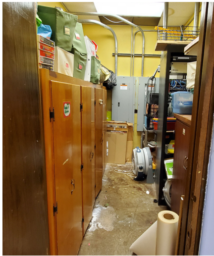
◀ This undersized TR houses non-IT items that inhibit front and rear rack access.
