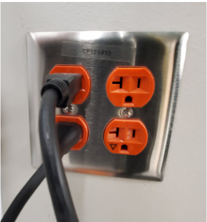
A dedicated electrical circuit with (2) 20A outlets (left) and an emergency generator outlet with proper labeling.
