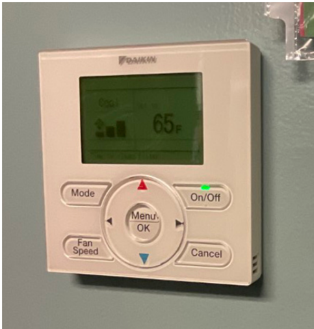
A standards-compliant, wall-mounted independent AC control unit in a TR.
