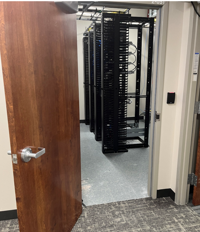
Entrance doors should swing out and have both card access and video surveillance.
