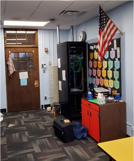
An IT equipment rack is installed in a space shared with a carpeted student resource room.
