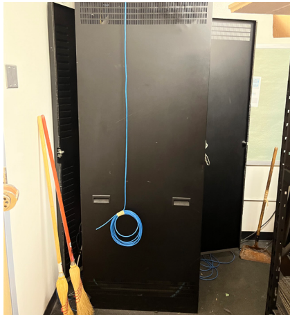
These TR racks lack adequate rear clearances; the one above also lacks sufficient lighting.
