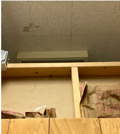
Walls should extend to the deck which is lacking in this TR.
