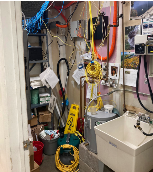
This TR is shared with a custodial closet with a utility sink that should not be in the space.
