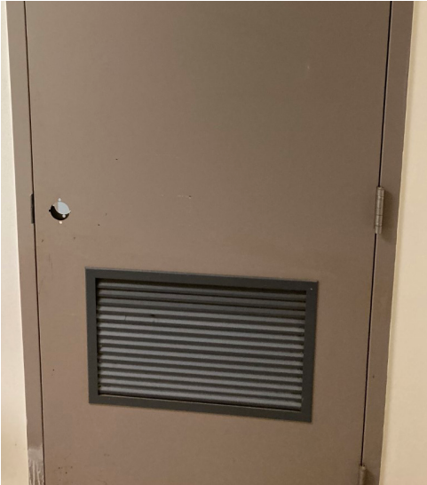
This TR exterior door lacks both a door knob and a locking mechanism.
