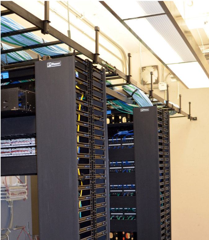
This TR has proper illumination as well as standards-compliant cable management, both overhead and at the racks.
