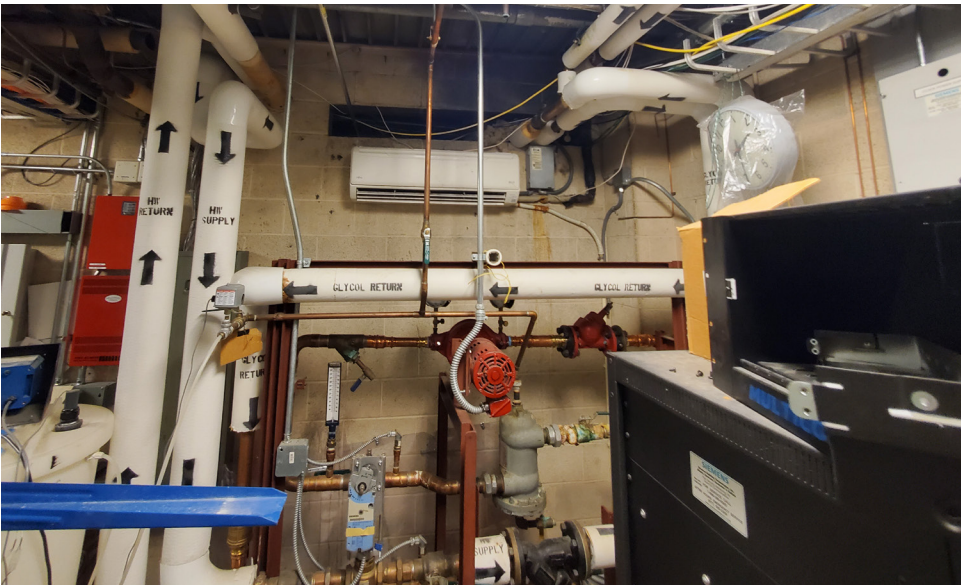
Pressurized water and glycol pipes are installed directly above and/or in close proximity to the IT equipment racks.
