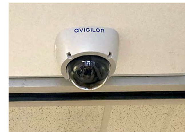
A ceiling-mounted surveillance camera can provide good security coverage of the front of the equipment rack in the space that is installed near the opposite wall.
