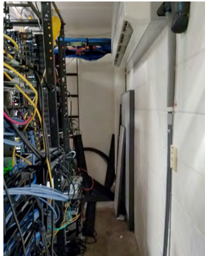
These TR racks lack adequate rear clearances; the one above also lacks sufficient lighting.
