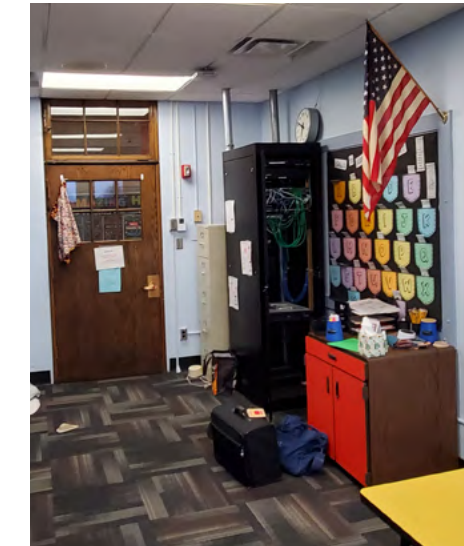
An IT equipment rack is installed in a space shared with a carpeted student resource room.
