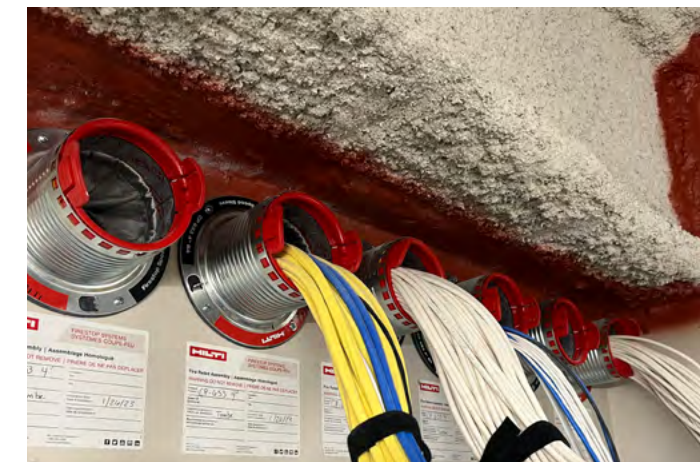
Below: Standards-compliant, fire-rated wall penetration assemblies.
