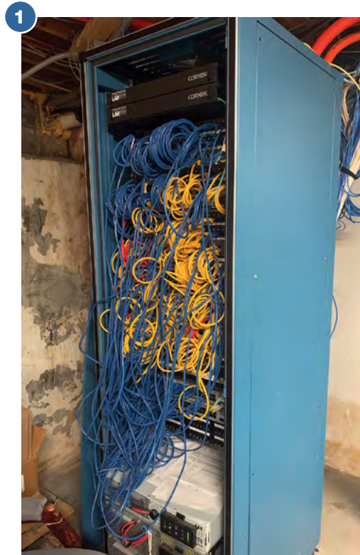
Photos, clockwise from top left: 1. The open rack is in an unsecured area that is shared with custodial items. 2. The space is below grade, a water pipe is installed directly over the rack, and cable management systems are lacking. 3. Conduits are filled beyond capacities. 4. There is a janitorial slop sink in the same space as the equipment.
